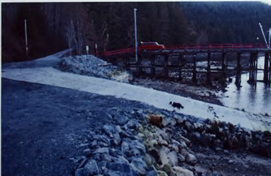
New boat launching ramp at Okeover.
